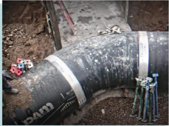
Fig. 4 / Assembly of cast iron pipes and accessories.
