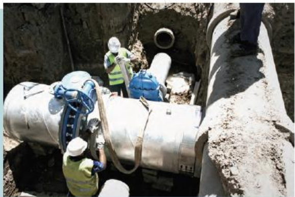
Fig. 6 / Assembly of pipes and accessories.
