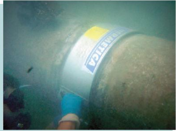
Fig. 2 / Underwater fitting. HERMETICA SF damp made of stainless steel AISI 316.
