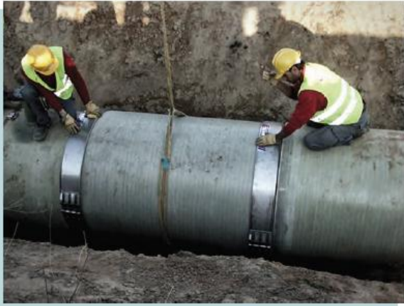
Fig. 1 / Fitting of large diameter GRP pipes.
