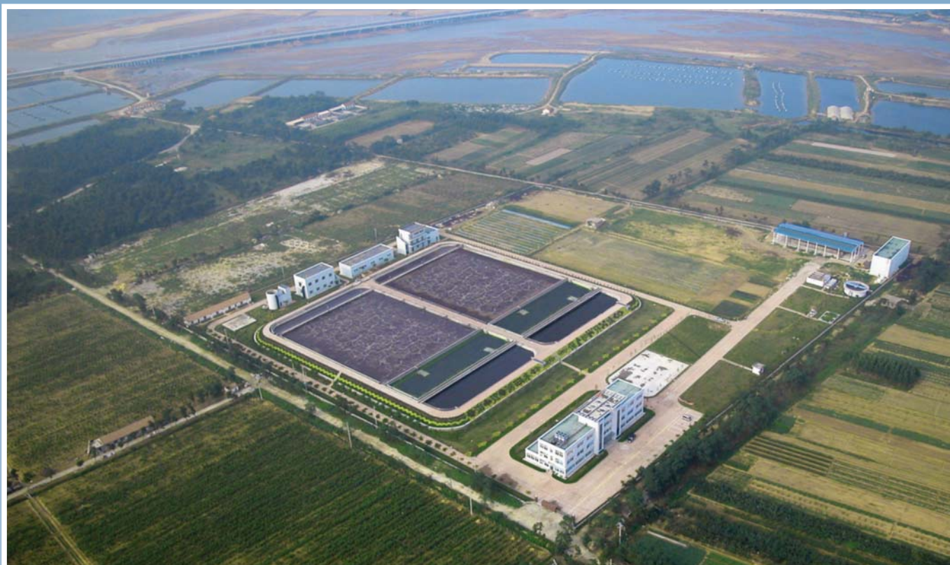
Municipality - waste water treatment plant, 40.000 m 3 /d - 200.000 p.e. 60
