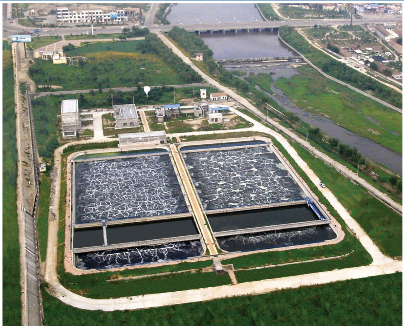
Municipality - waste water treatment plant 40.000 m 3 /d - 165.000 p.e. 60
