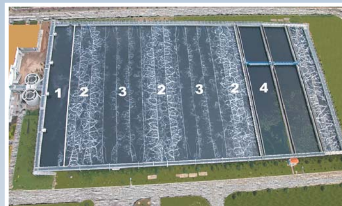
Municipality - waste water treatment plant 40.000 m 3 /d - 165.000 p.e. 90
