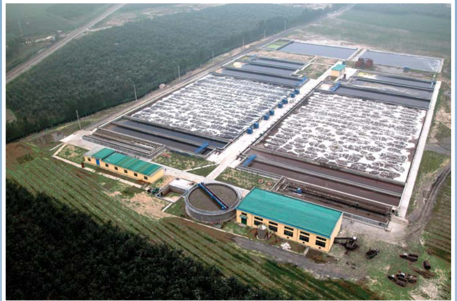
Wastewater treatment plant pulp industry 60.000 m 3 /d - 156.000 kg COD/d
