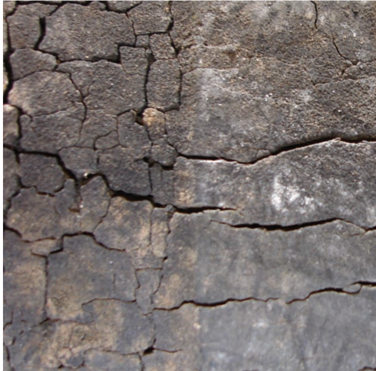
Porous surface caused by subjection to chemicals
